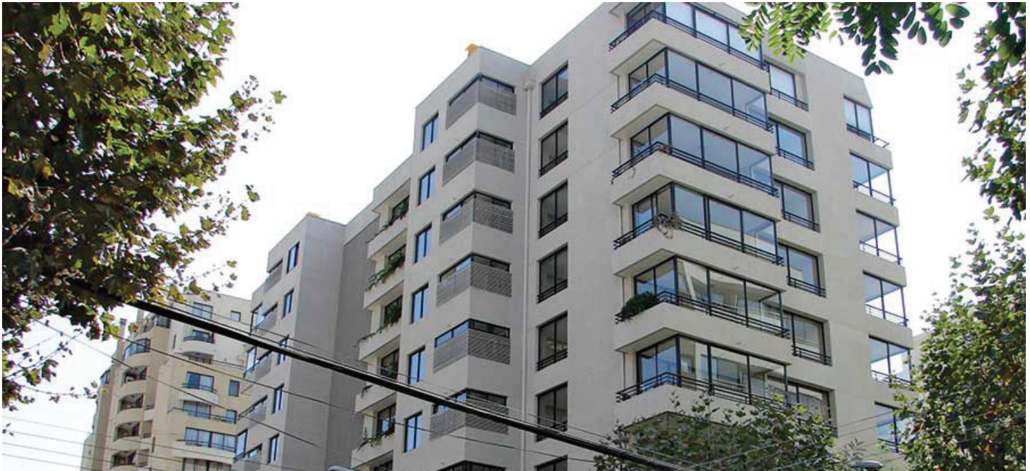
In Chile, a nonductile concrete building was damaged in an earthquake and then razed. Los Angeles' seismic retrofit law could apply to 1,200 buildings, but about half are no more than two stories. PHOTO COURTESY APPLIED TECHNOLOGY COUNCIL
